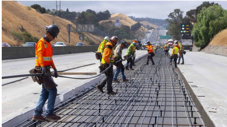
Pavement & Bridge Rehabilitation
