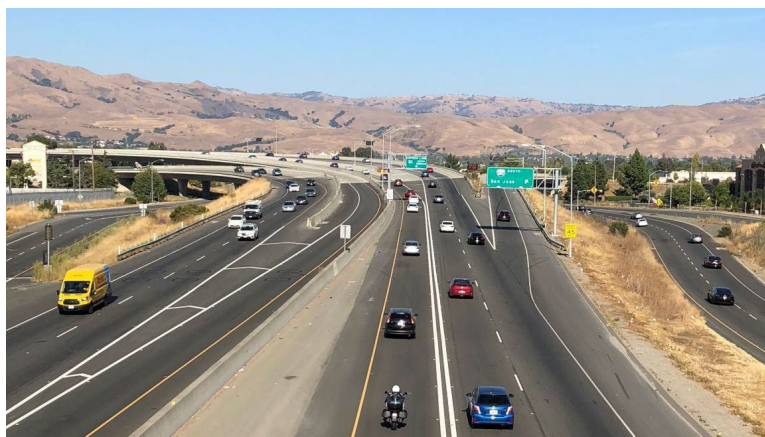
Bay Area: Express Lane Corridors Limited express bus utilization
