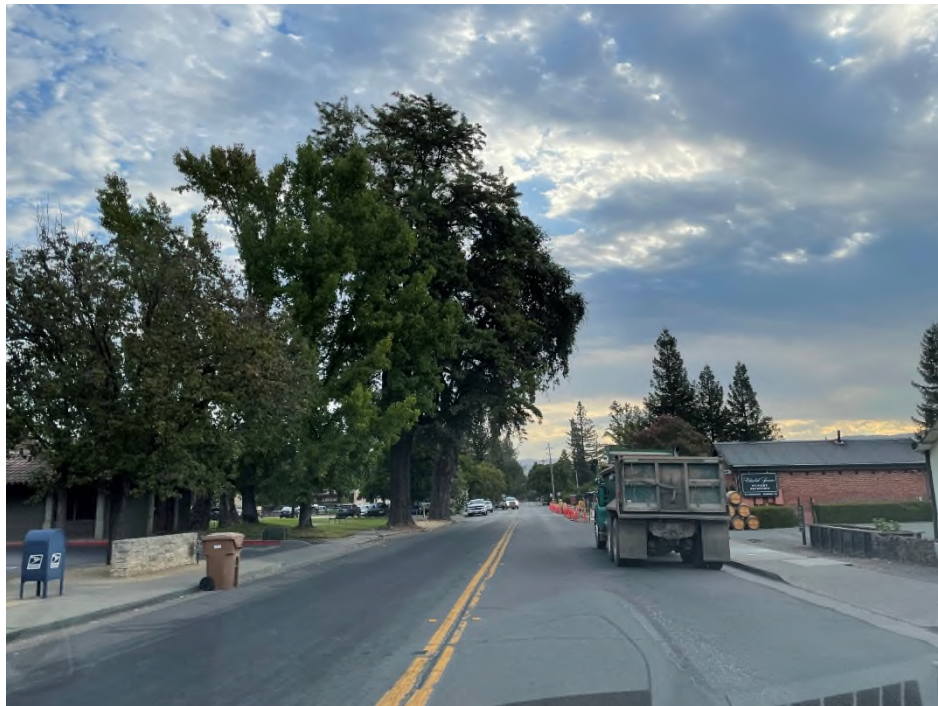
Photo 6: Project site, facing northeast at Rutherford Rd.
