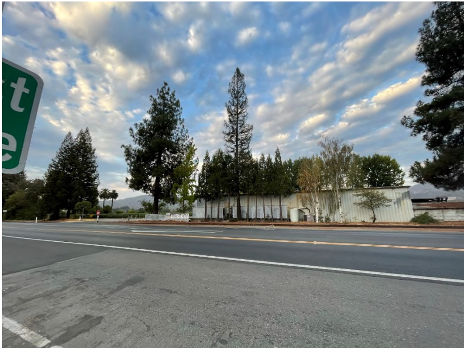
Photo 2: Project site, facing west at Oakville Pump Service facility.
