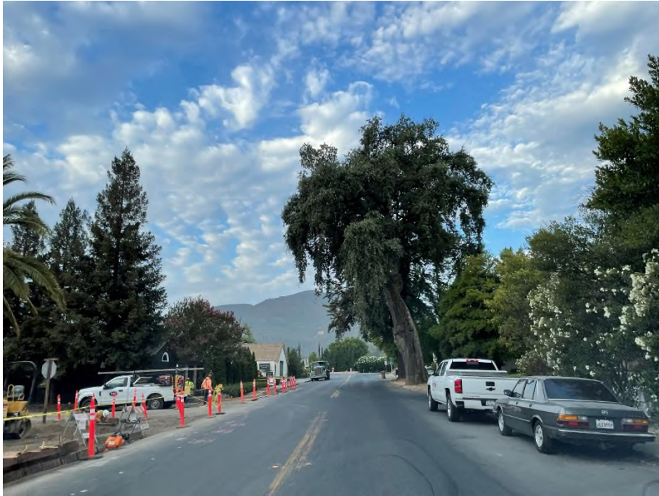
Photo 7: Project site, facing southwest at Rutherford Rd.
