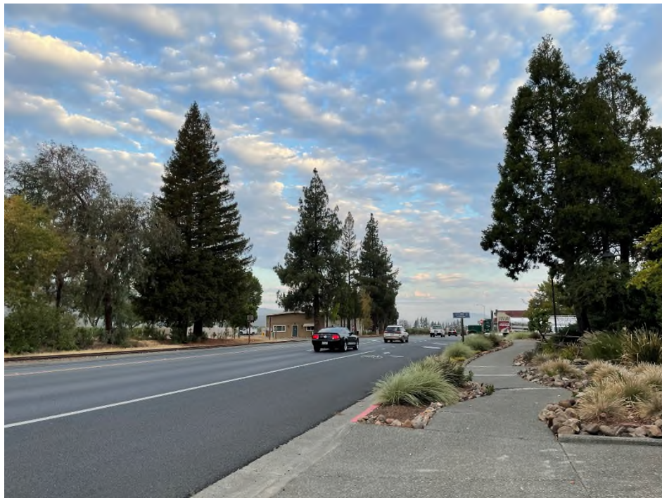
Photo 6: Project site, facing northwest toward SR-29 and Oakville Cross Rd intersection.
