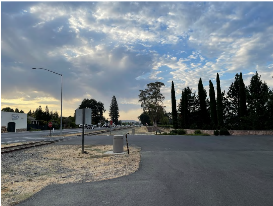
Photo 4: Project site, facing south at intersection of SR-29 and Rutherford Rd along railroad right of way.
