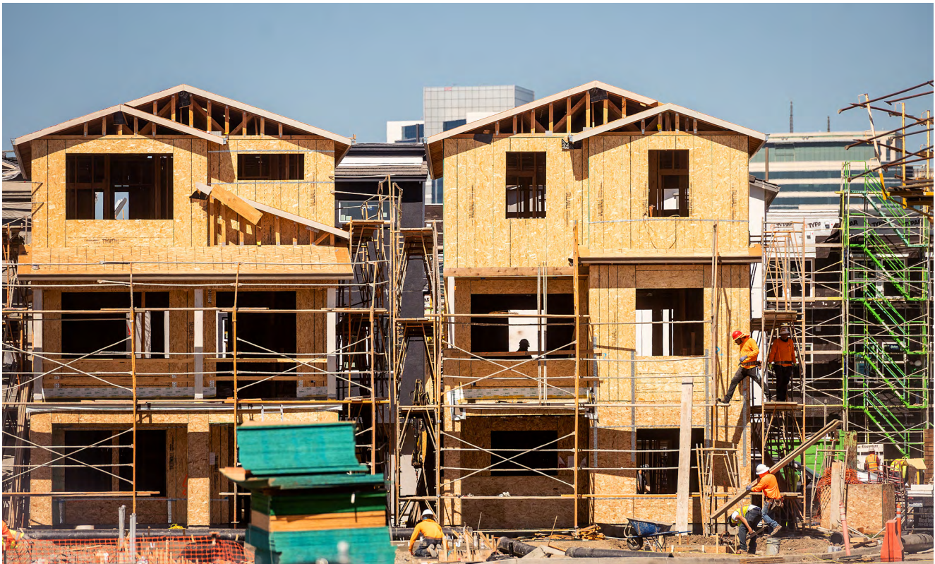
Multifamily home construction, Santa Clara County Photo: Noah Berger
