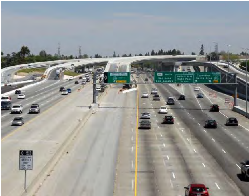
Pictured: 101/SR85 interchange in Mountain View
