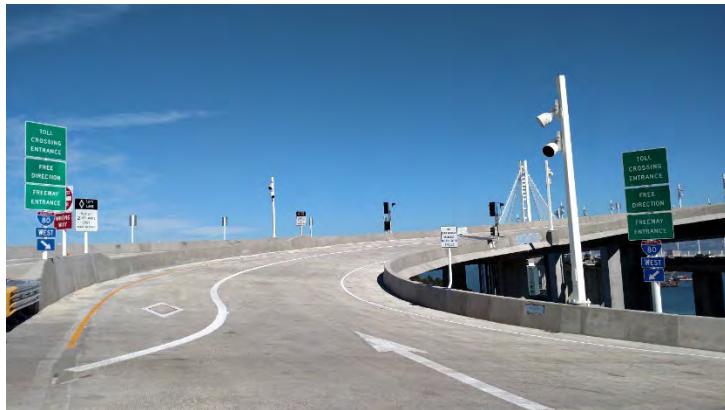
Pictured: WB I-80 on- and off-ramps that connect Yerba Buena Island and Treasure Island to the eastern span of the Bay Bridge.
