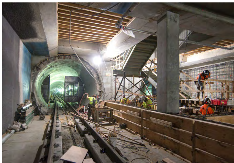
Pictured: Construction of SFMTA's Central Subway Project
