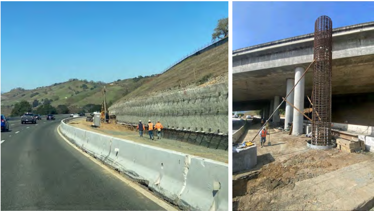
Pictured: I-680/84 Interchange Improvements project under construction
