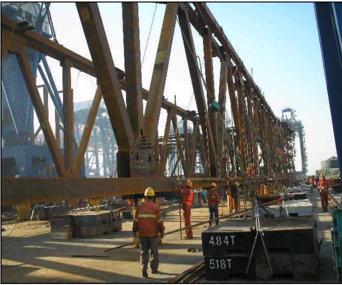
Temporary Support Truss Being Fabricated at ZPMC
