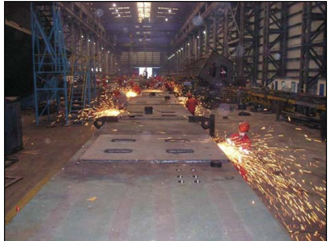
Welding Doublers Plates onto Tower Lift 1 North Shaft Skin A
