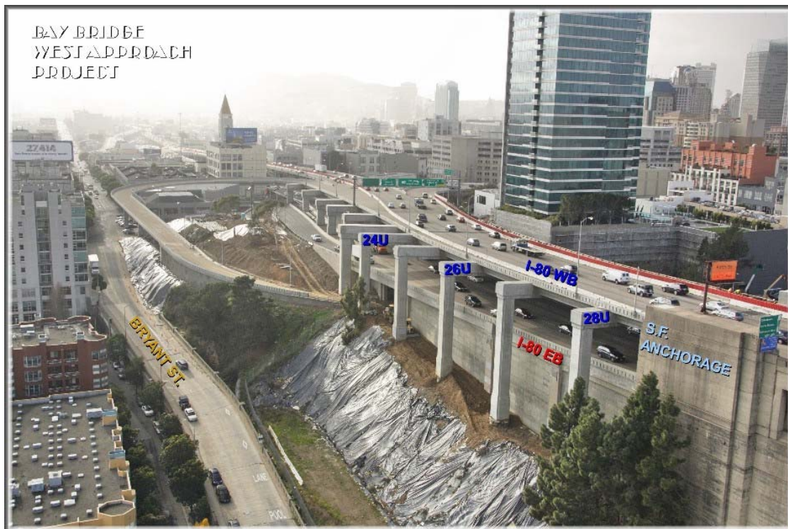
West Approach Project Progress
