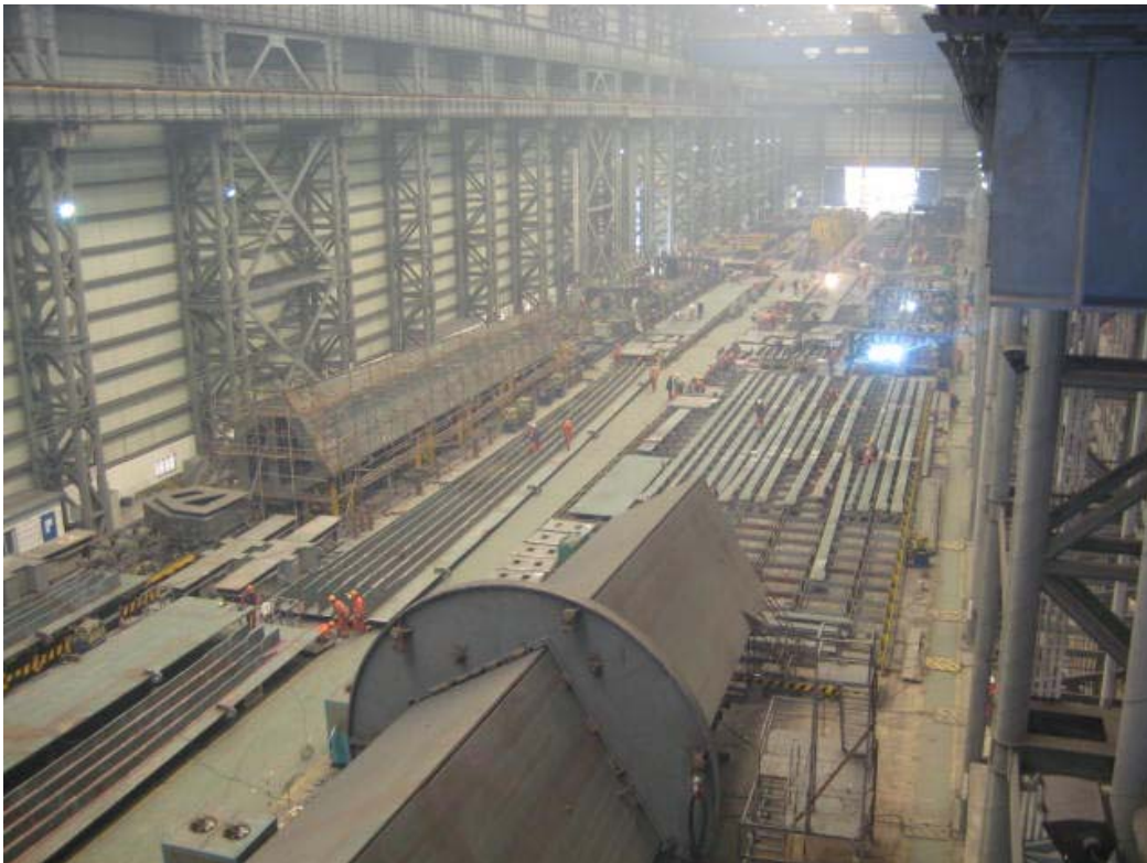
Tower Lift Shaft Fabrication
