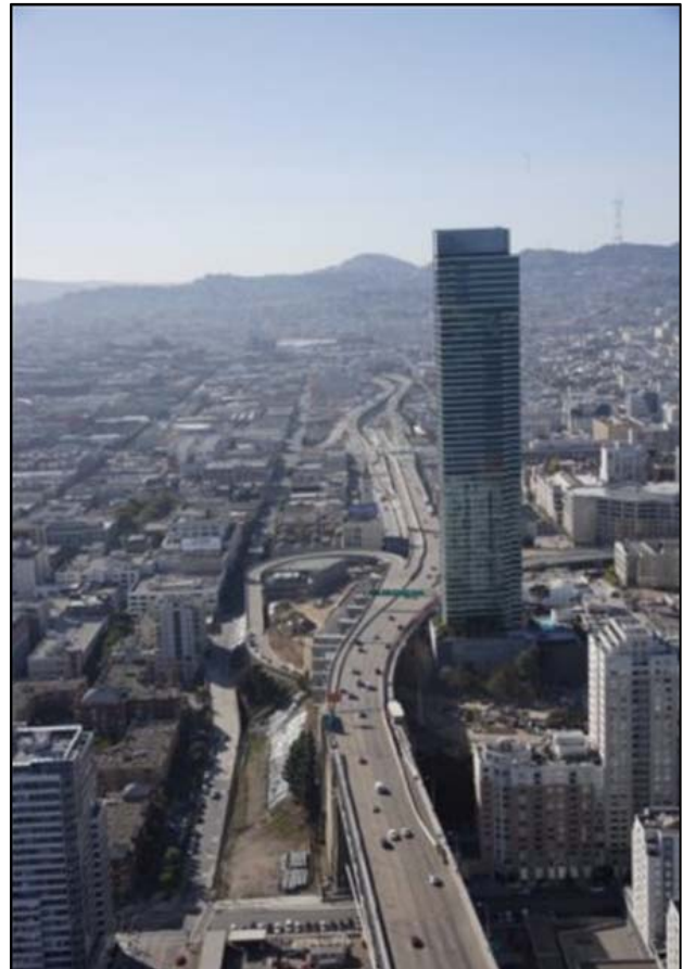
The West Approach Aerial View
