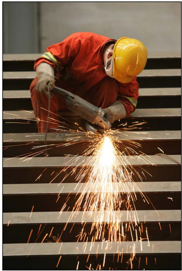
Orthotropic Box Girder (OBG) Side Panel Grinding
