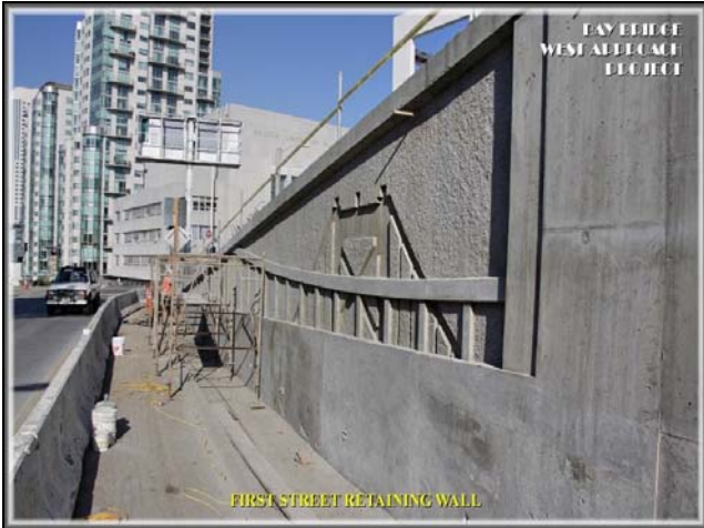
First Street Retaining Wall
