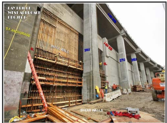
Infill Wall and Shear Walls under I-80 Eastbound
