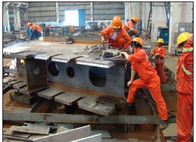
Tower Double Diaphragm Outline Beveled after Machine Milling
