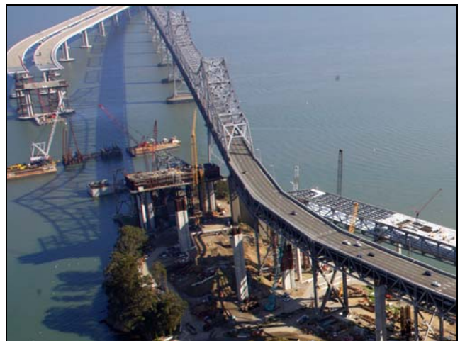
Aerial View of Yerba Buena Island Transition Structures (YBITS)
