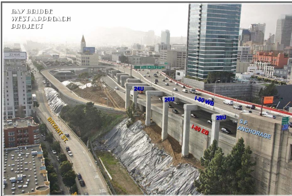
West Approach Replacement Project Aerial View
