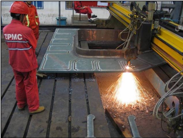
Main Tower Diaphragm Plate Cutting
