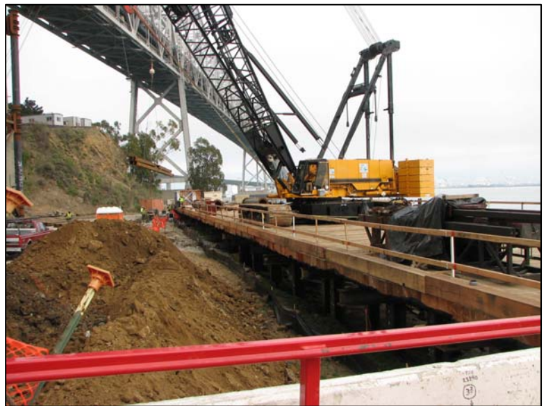
East Tie-in Temporary Crane Runway Platform
