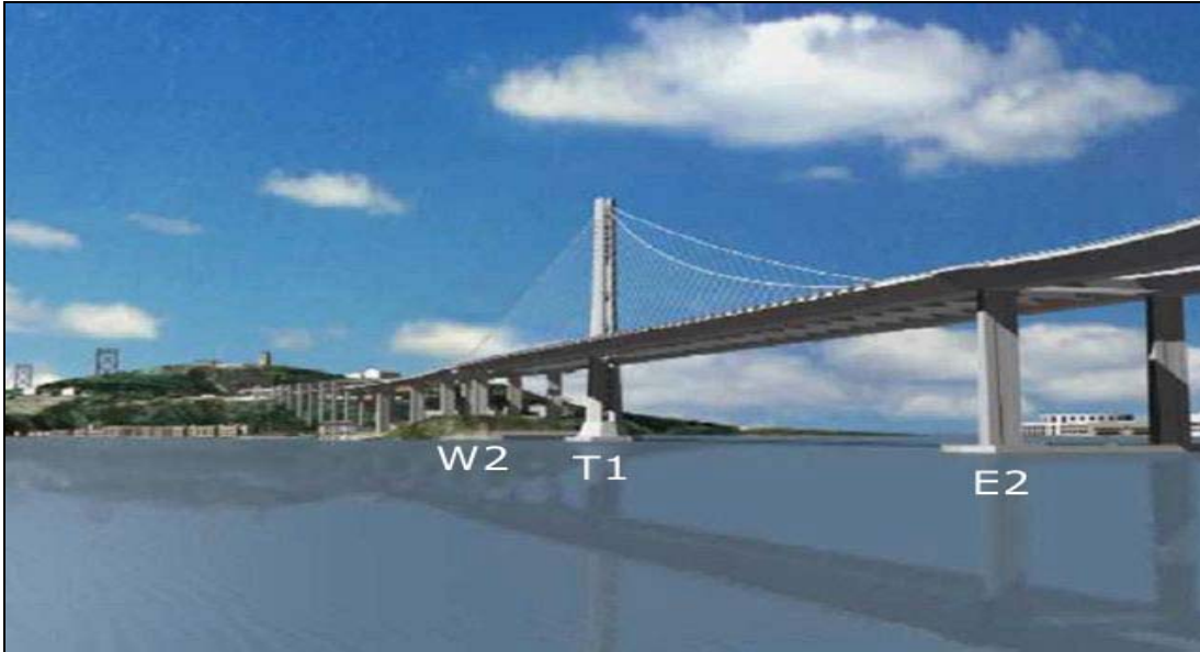
T1 = Foundation for the 530-foot steel tower E2 = Eastern Support of the suspension roadway W2 = Western Support of the suspension roadway
