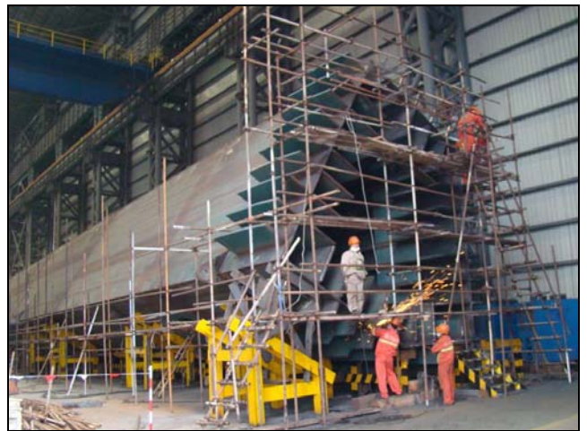
Welding Doublers Plates onto Tower Lift 1 North Shaft Skin A
