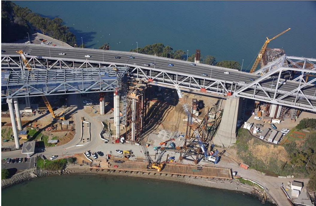
East Tie-In (ETI) Skid Bent System Erection
