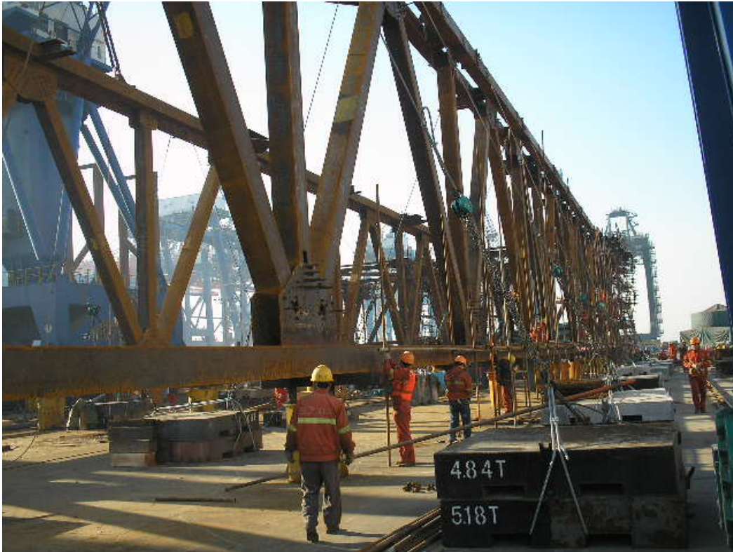
Temporary Tower Truss Fabrication at ZPMC
