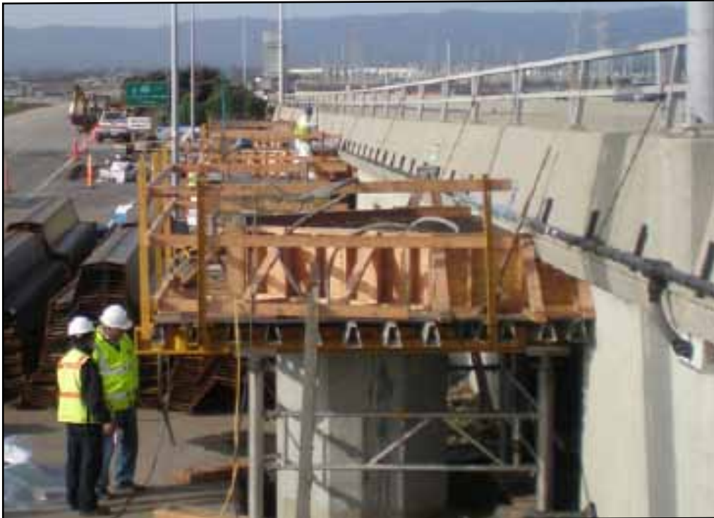
Series of Bent Cap Extensions Ready for Casting of Concrete
