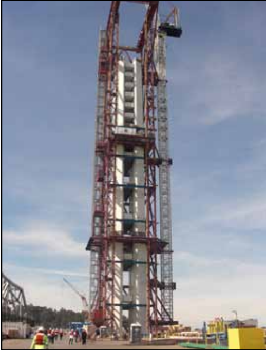
Tower Showing the Fourth Lift Complete on left and a Close up on right of the Tower with the Newly Installed Tower Bracing Architectural Facades
