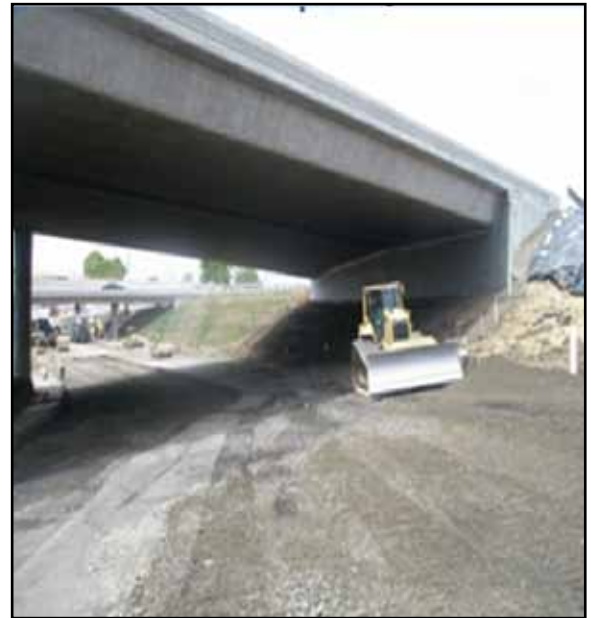
Gore Area Concrete Paving in Progress and South-bound 880
