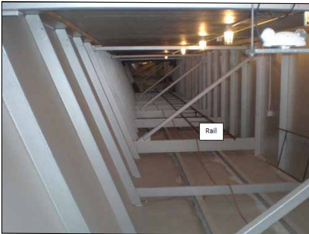
Rail for Material Transporter Supported at Cross Frames within Box Girder
