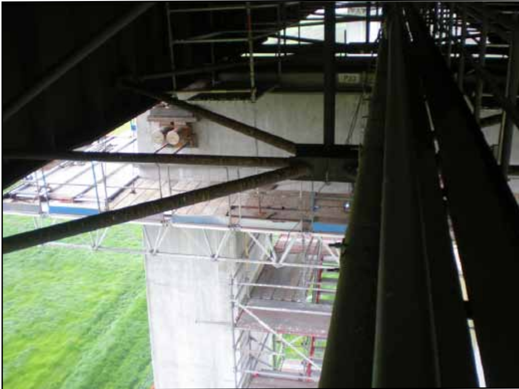
Jacking Pins at Pier 33
