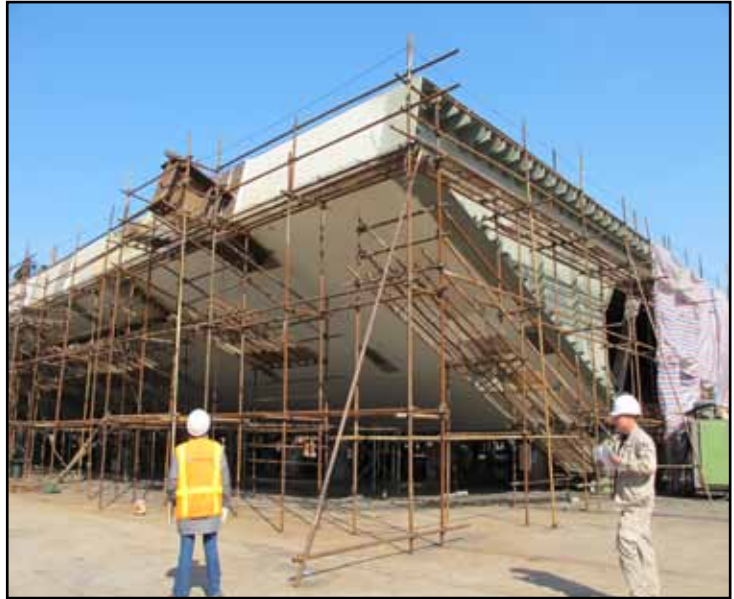
Roadway Box 12 in Trial Assembly
