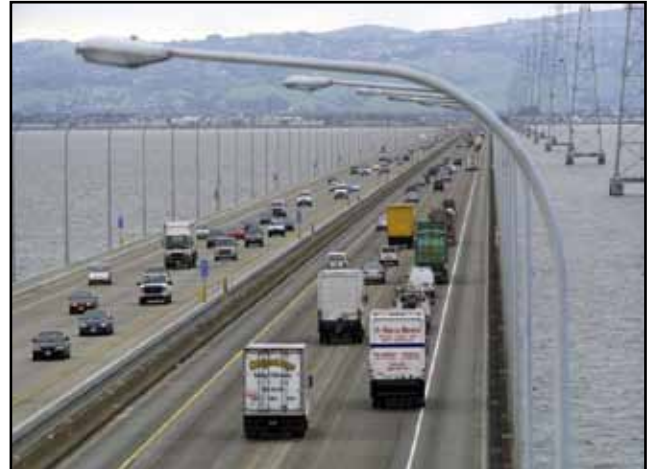
Widening of the San Mateo-Hayward Bridge Trestle on Left
