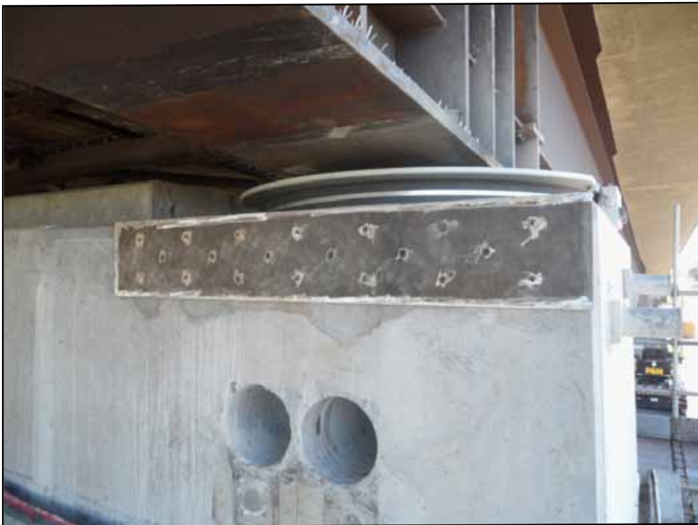
Sole Plate Prior to Stainless Steel Sheet Installation
