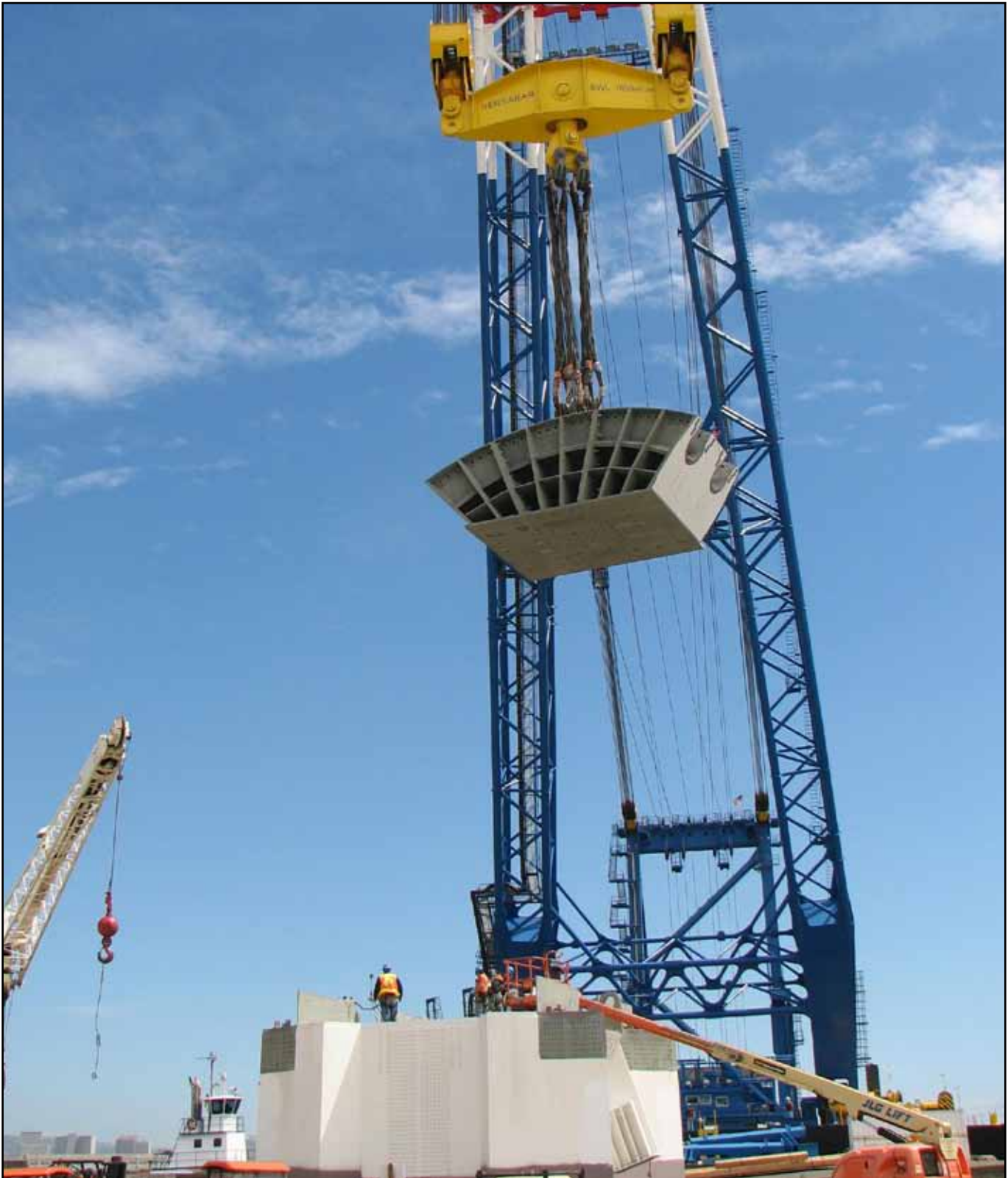
Tower Saddle Being Lowered onto the Grillage
