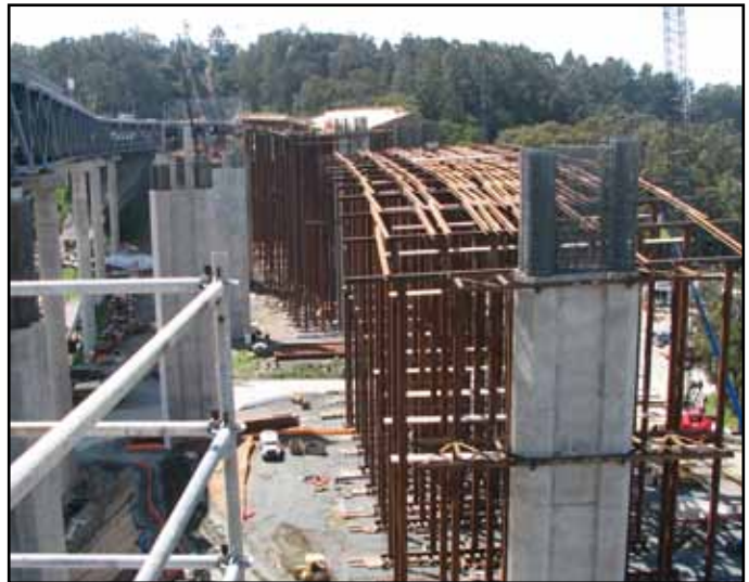
YBITS #1 Westbound Frame 2 Falsework
