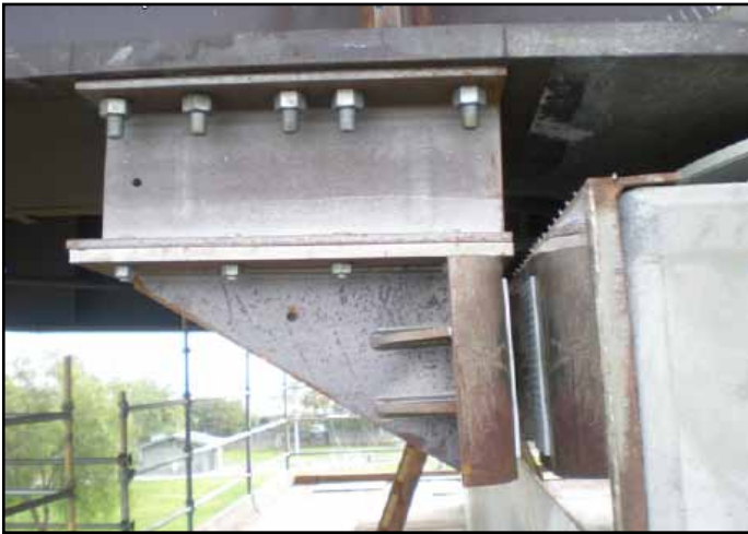
Antioch Bridge - Restrainer Bracket at Pier 5
