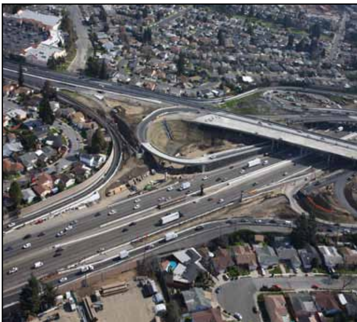
Aerial View of Construction Progress
