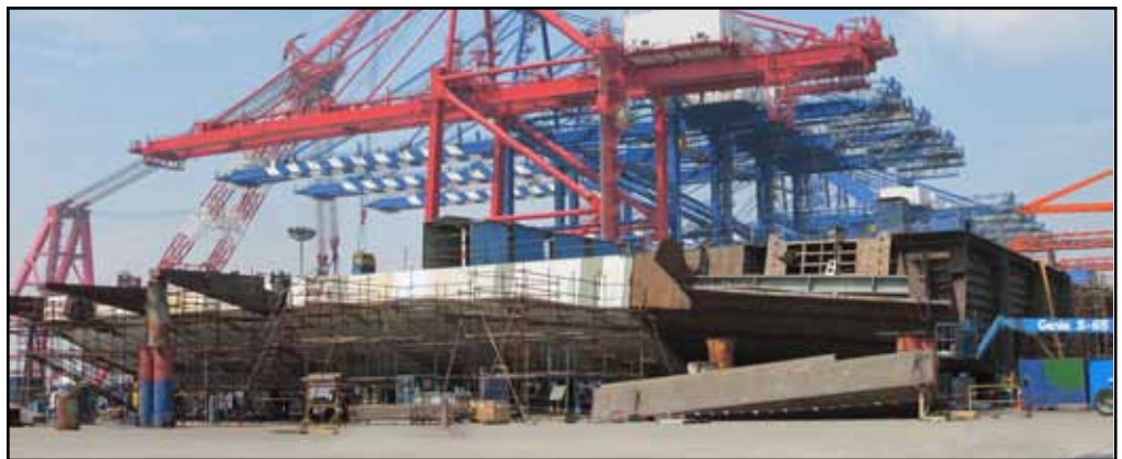
Roadway Box 12 and Segment 13 A in Trial Assembly
