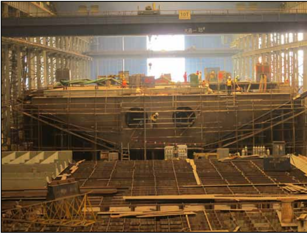
Roadway Box 14 East
