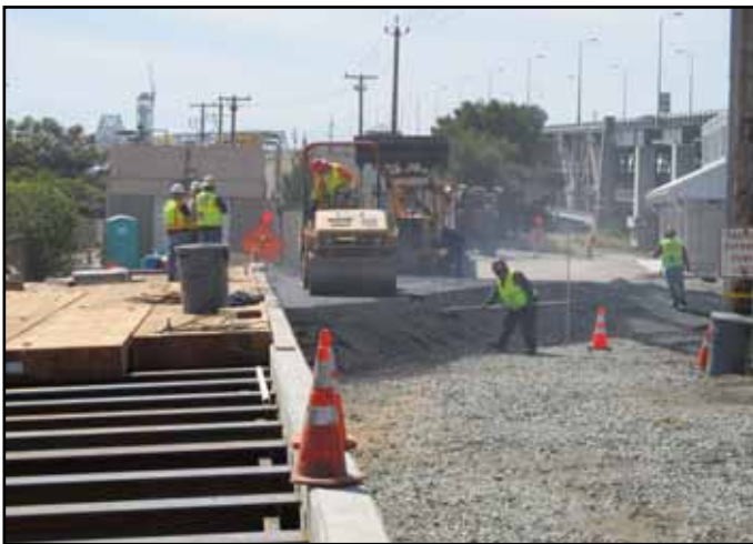
Oakland Detour EBMUD Outfall Bridge Planks & Structural Steel Support Installed
