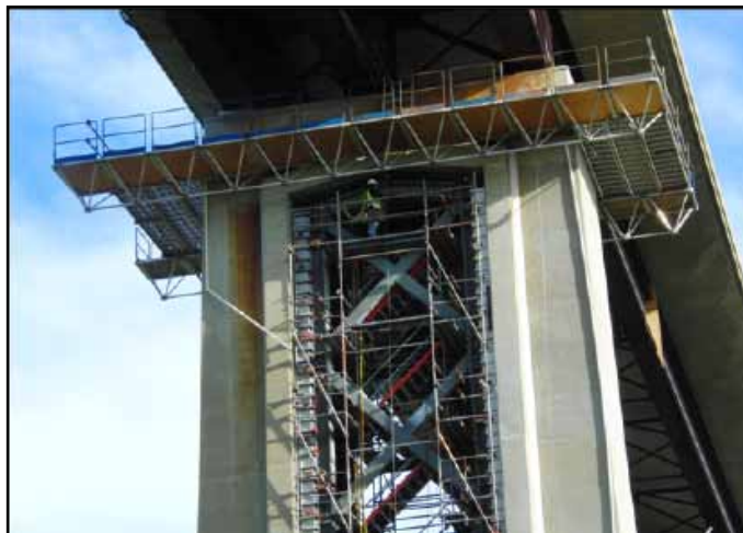
Forms Installed to Upper Chord at Pier 30 of Antioch Bridge
