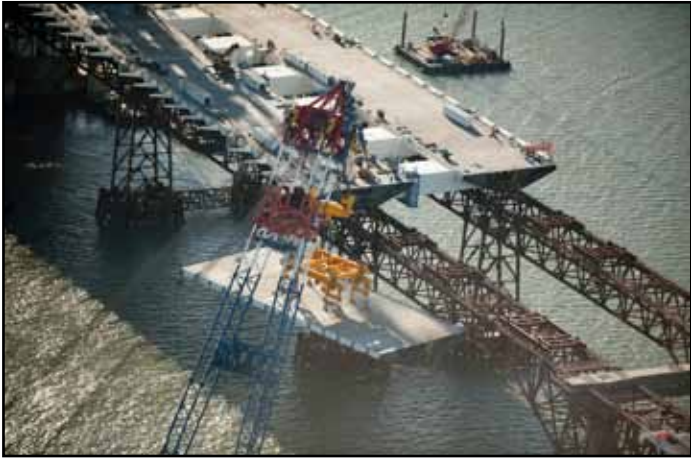
Shear-Leg Crane Barge in Process of Lifting Roadway Box 11 E
