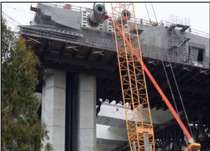
Pier W2 and Hinge K and West Deviation Saddle Installed
