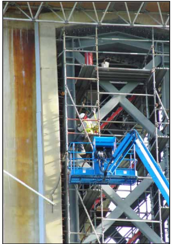
Bolting at Cross Frame Connection at Pier 31
