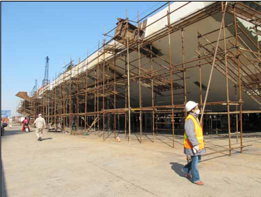
Roadway Box 12 and 13A Undergoing Trial Assembly
