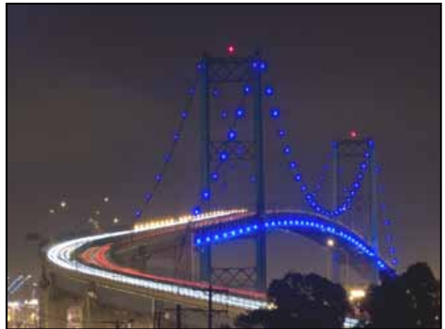
Los Angeles-Vincent Thomas Bridge
