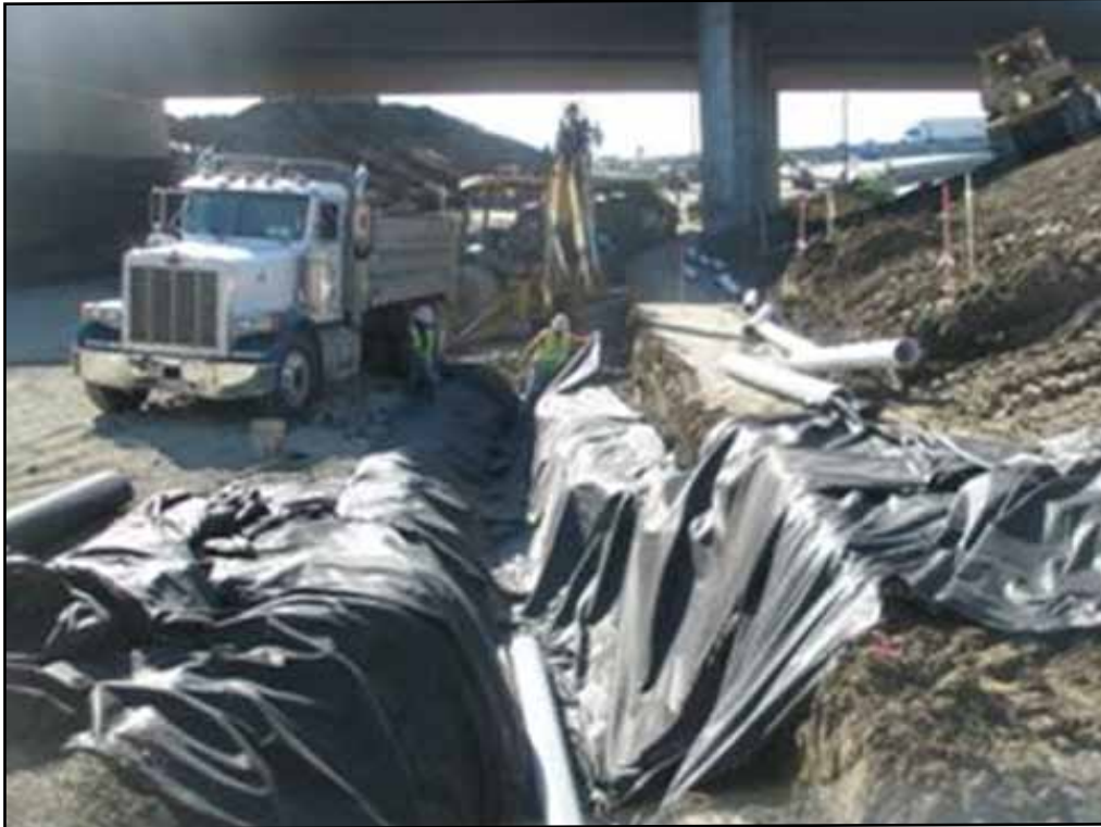
Under Drain Installation in Progress along J-7 Line
