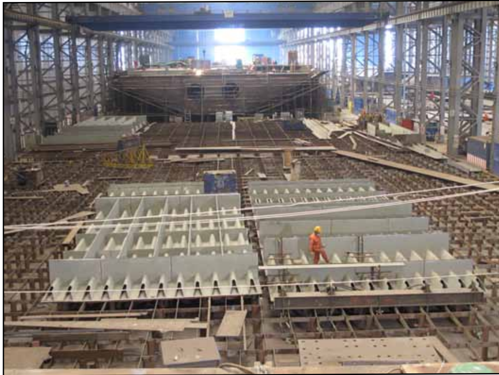
Deck Panels for Roadway Box 14 - Last Deck Panels for Entire SAS Project
