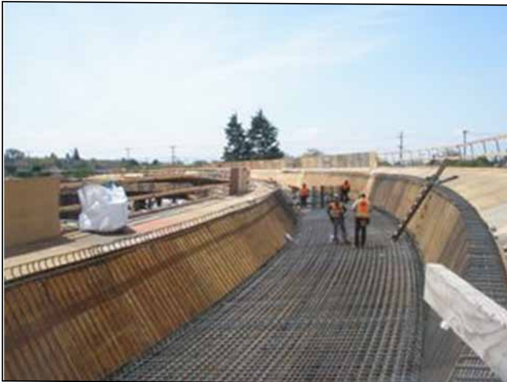
WSCONN Bridge Construction in Progress
