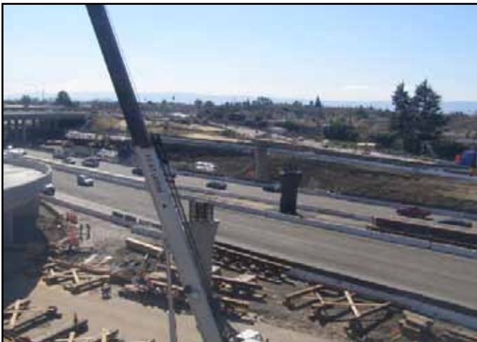
92/880 NWCONN Bridge Construction
