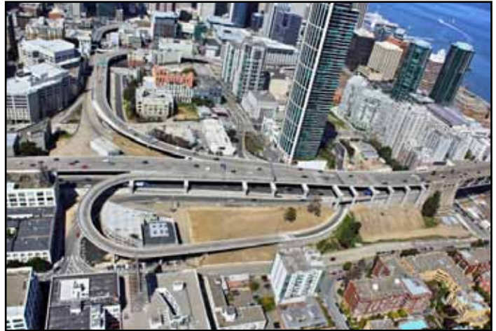
West Approach Overview
