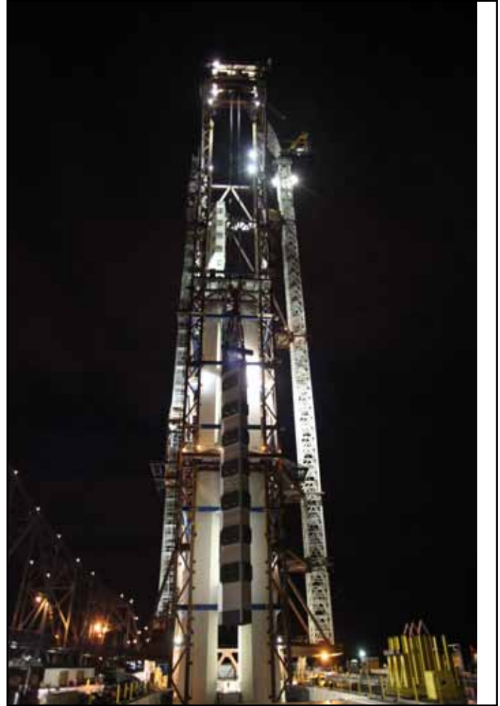
Tower Lift 4 Leg 2 Being Erected
