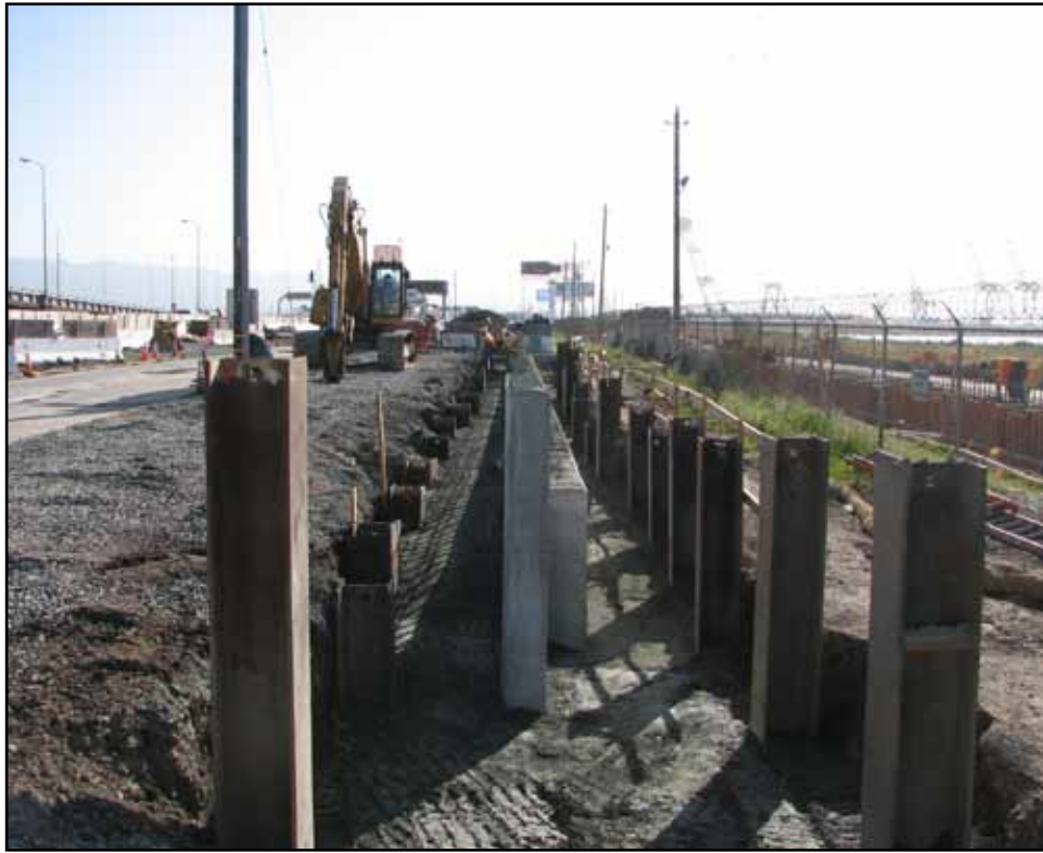
East Bay Municipal Utility District (EBMUD) Overcrossing North Abutment Wall
