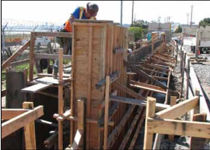
Oakland Detour North Abutment Formwork
