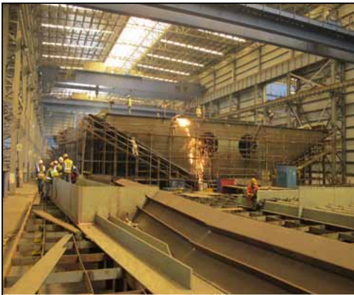
Roadway Box 14 East with Center Deck Panel in Place
