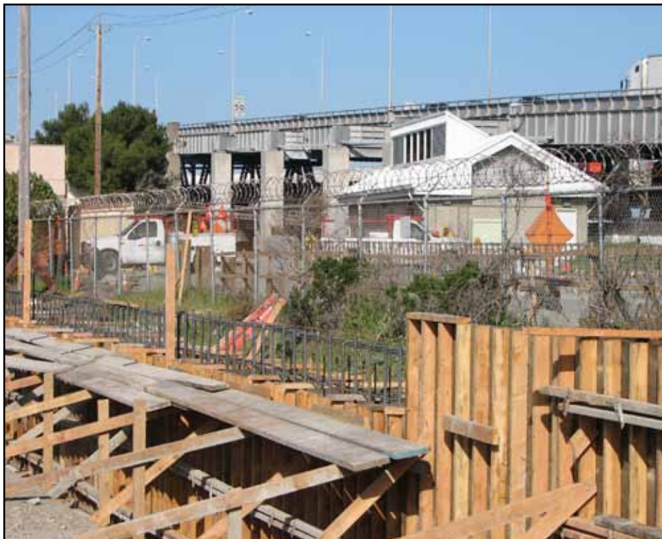
East Bay Municipal Utility District (EBMUD) Overcrossing Abutment Walls
