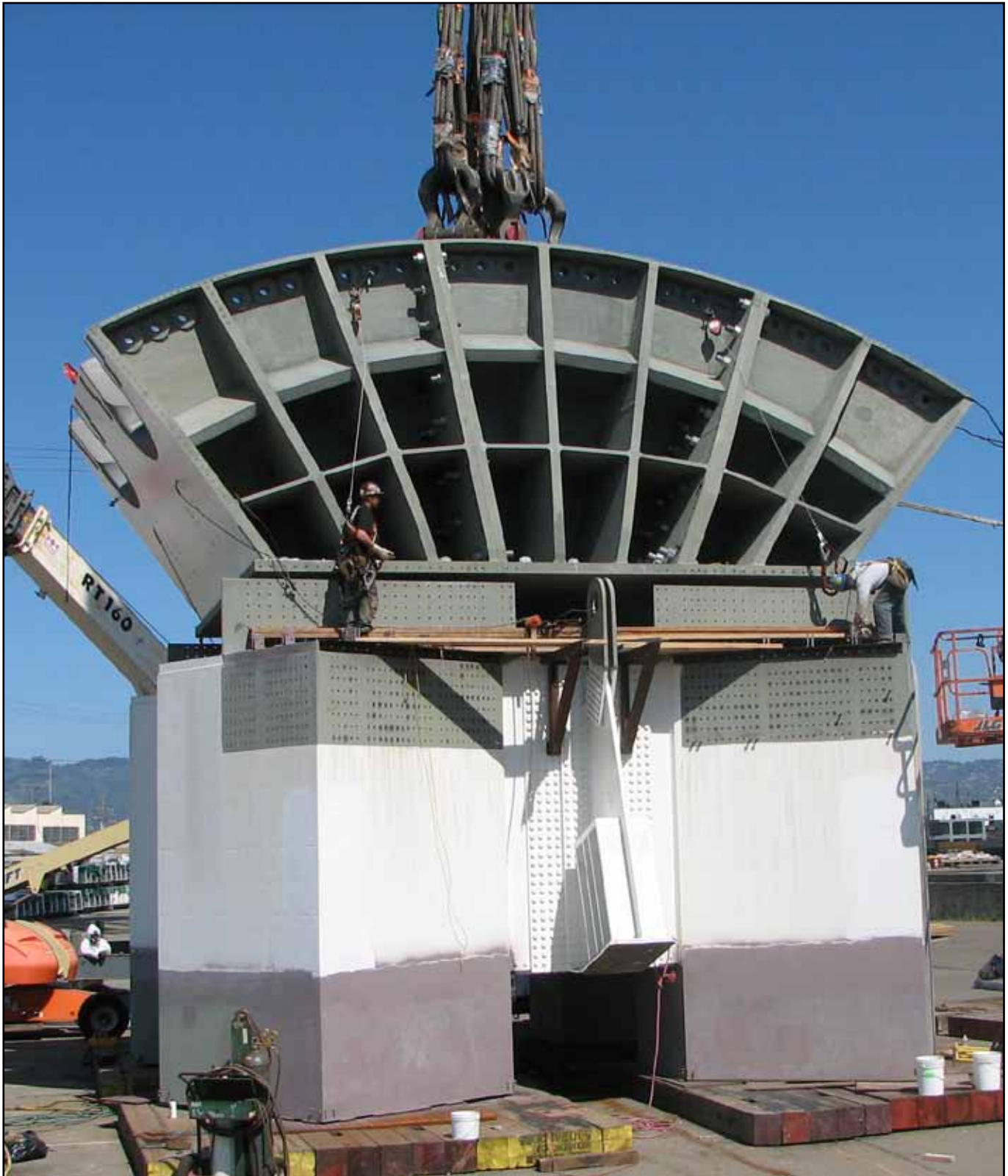
Tower Saddle Being Installed on Grillage
