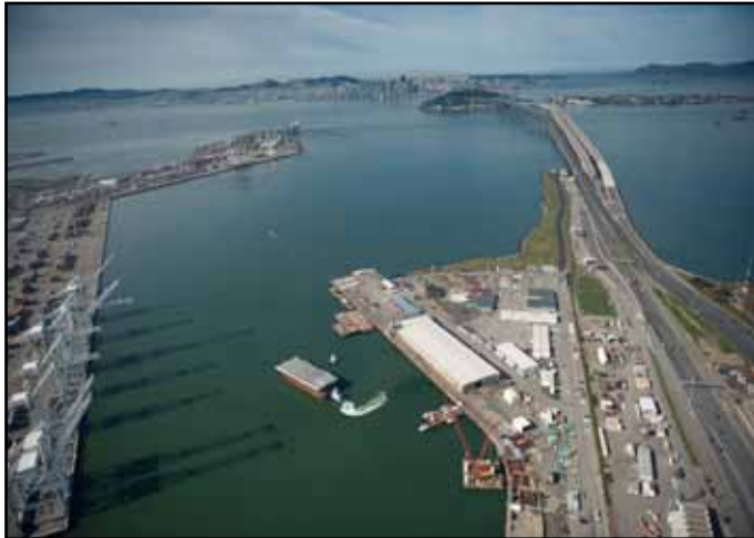
Roadway Box 11 Being Transported from Pier 7 in Oakland to the Shear-Leg Barge Crane for Placement
