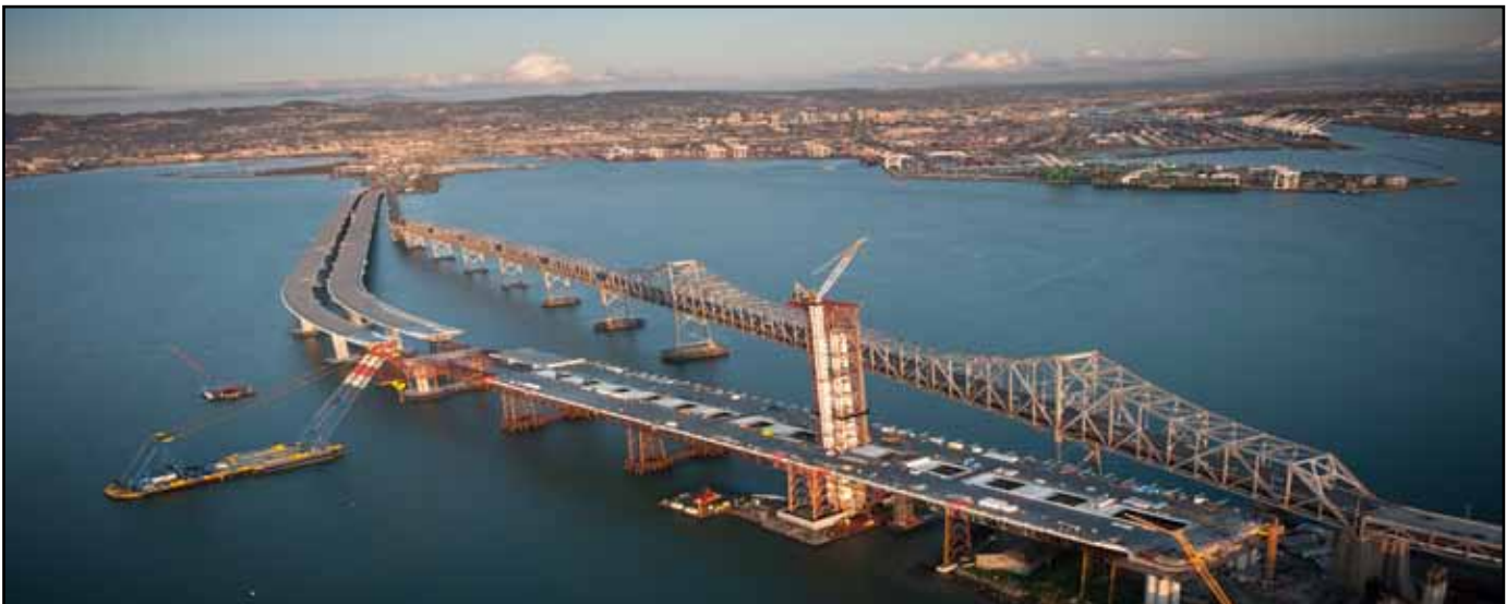
Aerial View of Current Progress on the Self-Anchored Suspension Bridge
