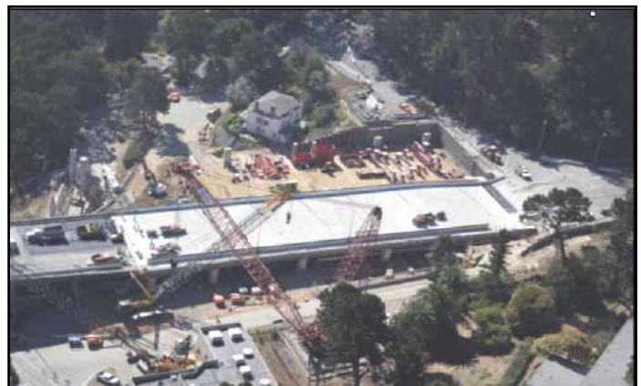
West Tie-In Phase #1 Rolled in on Labor Day Weekend 2007
