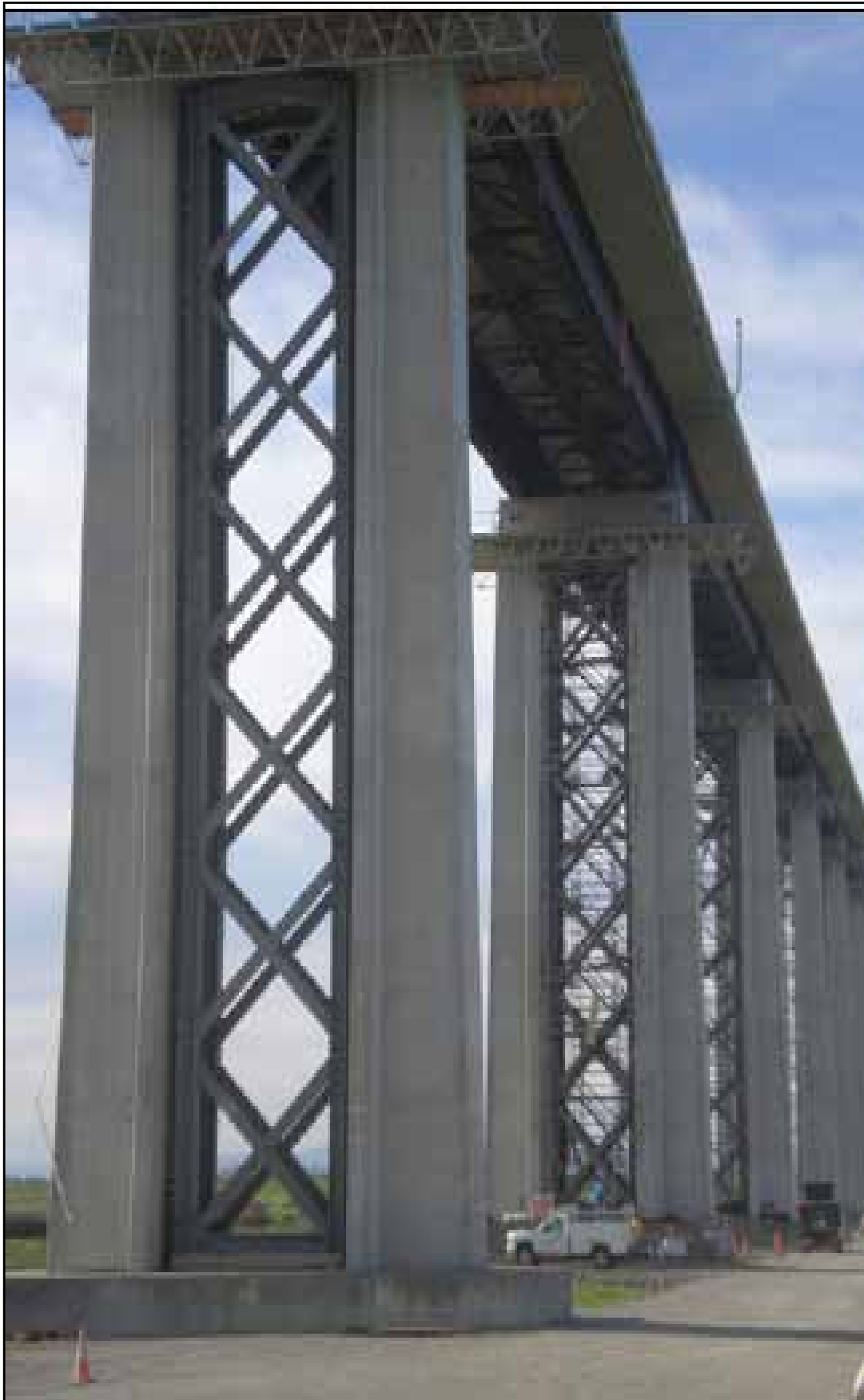
Piers 29, 30 and 31 at Different Stages of Cross-Brace Installation
