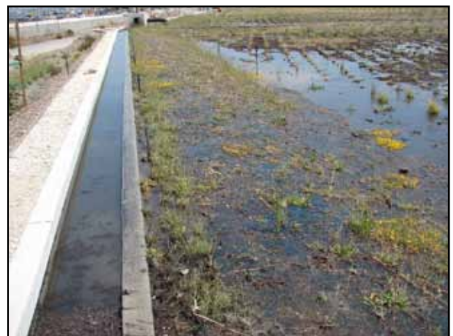
Stormwater Retention Basin
