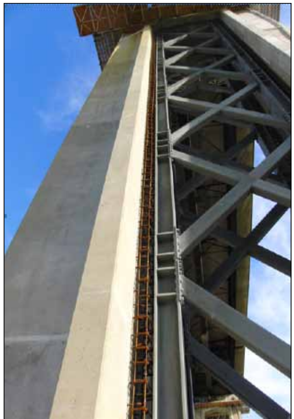
Reinforcing Steel Placed for Concrete Pedestal at Cross Frames at Pier 29
