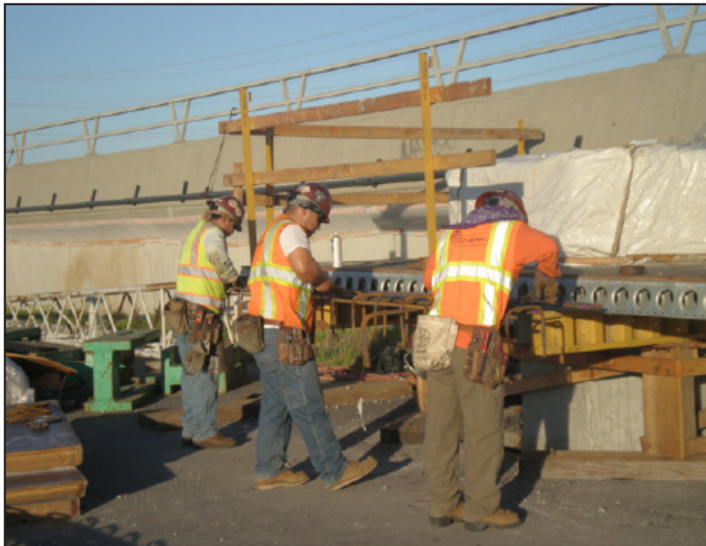
Iron Workers Fabricating Reinforcing Cages
