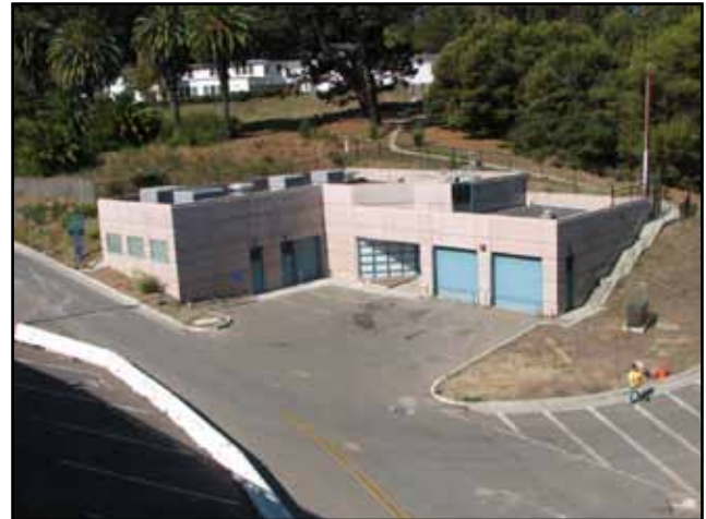
New YBI Electrical Substation
