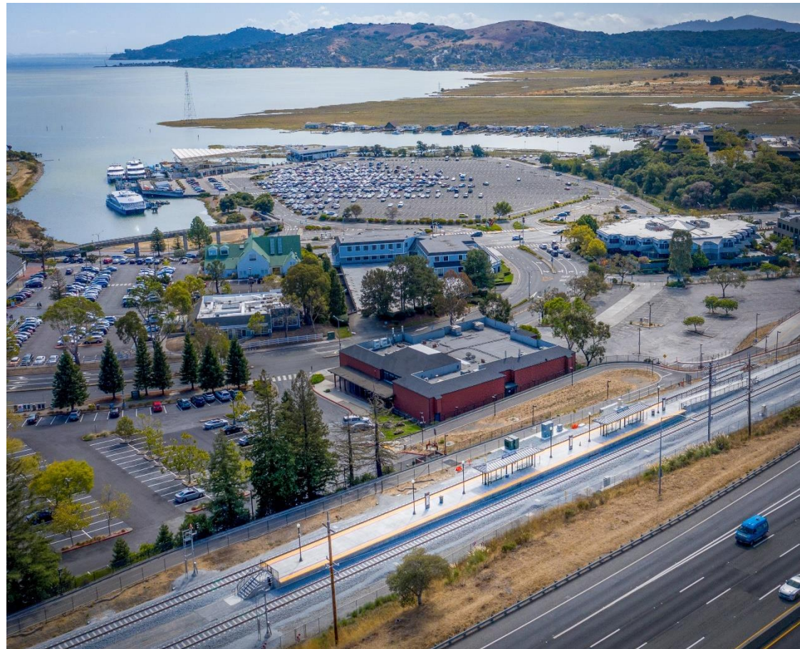
Similar to the Larkspur SMART Station and Ferry Terminal hub area, mobility hubs dispersed across a large portion of land area will require coordinated governance and operations.
