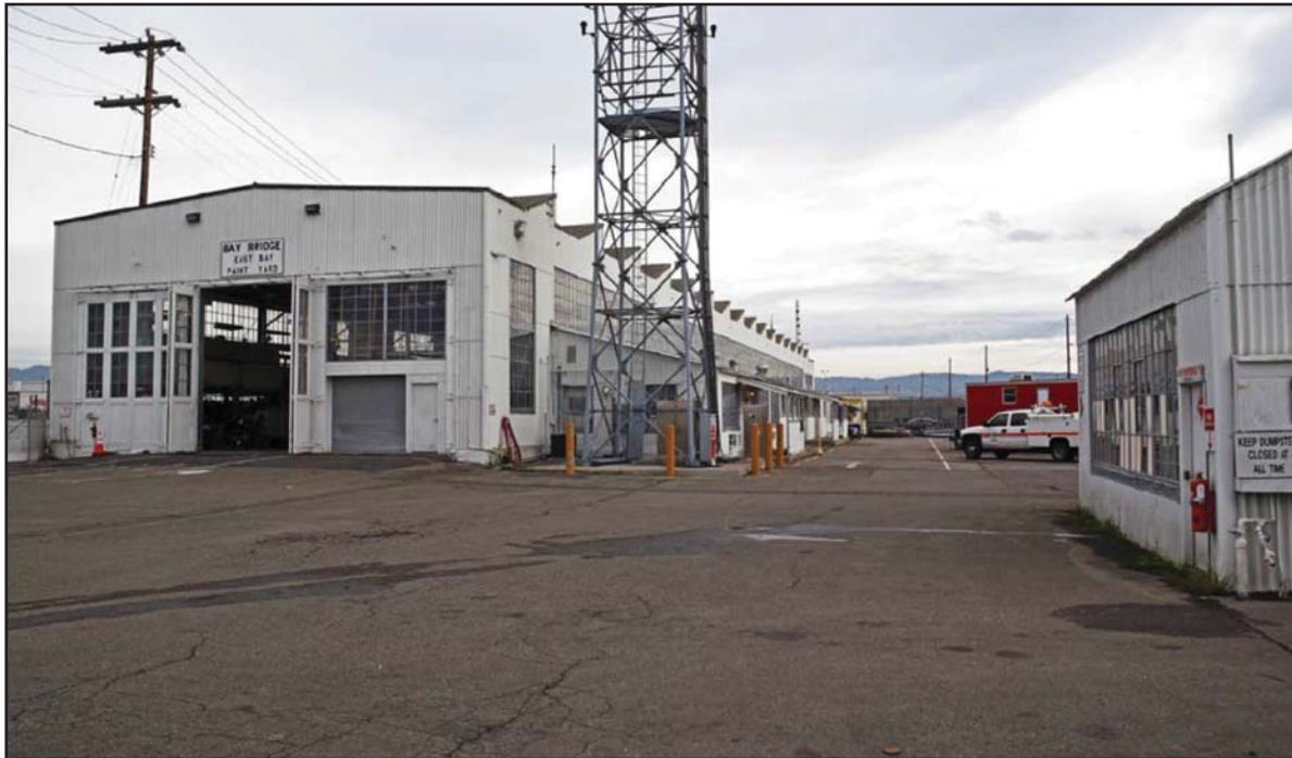
Existing Conditions (12/8/2014), from Portside VAU looking east toward the IERBYs Building. (Note: as part of a separate project, the IERBYs building was seismically retrofitted and a parking lot was constructed south of the building after this photo was taken.)
