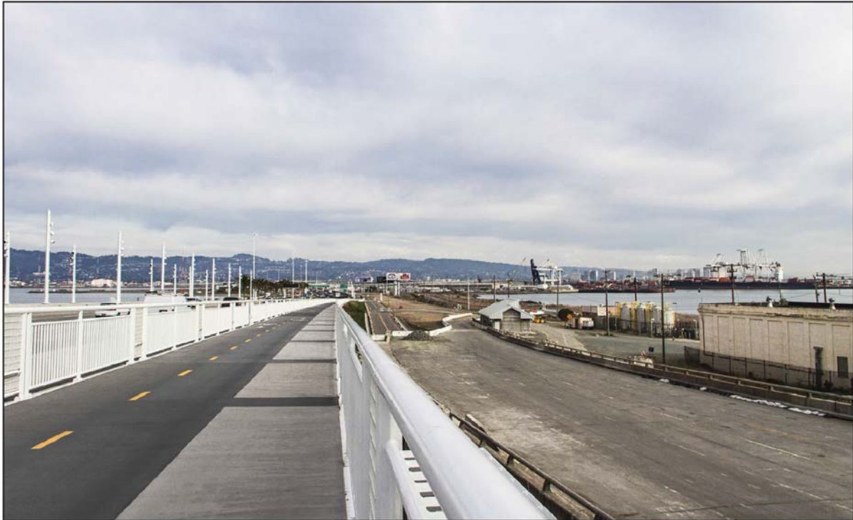
Existing Conditions (11/18/2014), from Bay Bridge Trail looking east toward the Portside VAU.
