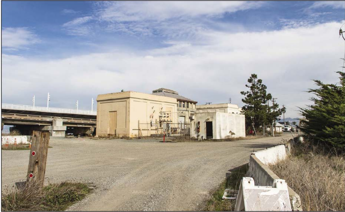
Existing Conditions (11/18/2014), from Portside VAU looking east toward the Historical Key Building.
