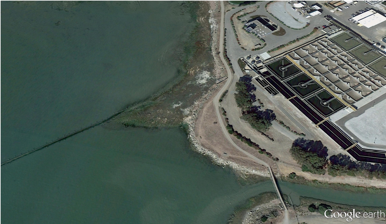
Figure 2.11 Riprap Protection for Wastewater Treatment Plant, San Leandro (Wetlands and Tidal Flats Outboard)
