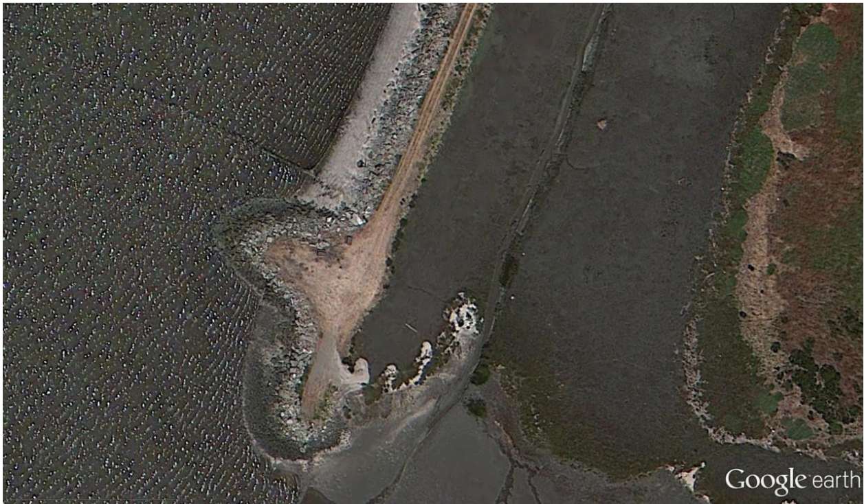
Figure 2.14 Nonengineered Berm with Riprap-Protecting Tidal Marsh from Wave Erosion, Hayward (see Hayward Marsh Figure 2.17 below under “Wetlands”)
