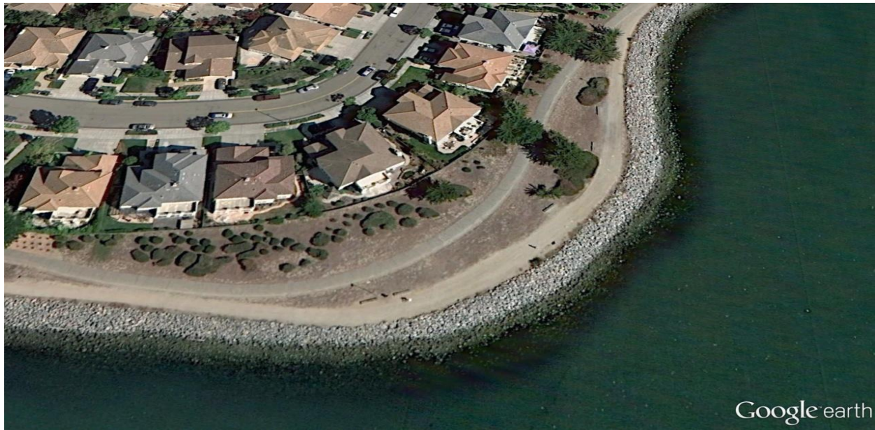
Figure 2.8 Revetment, Shoreline Park, Alameda
