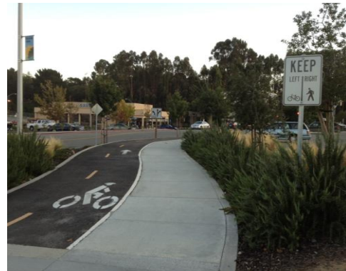
Coffey lane extension pedestrian/bicycle path
