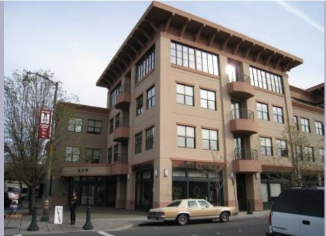
Offices over retail/service
