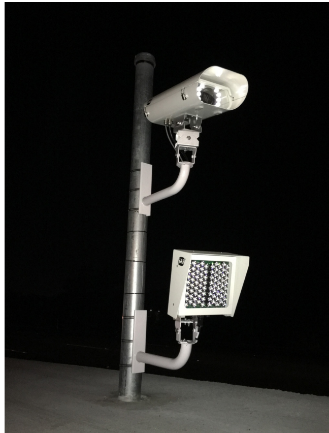
Violation camera for the toll system. (See additional construction photographs on pages 17-18)
