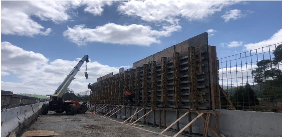
Construction of forms for sound wall on I-680 in Alamo/Walnut Creek
