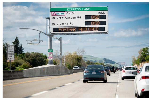
Overhead pricing sign on the I-680 Express Lanes
