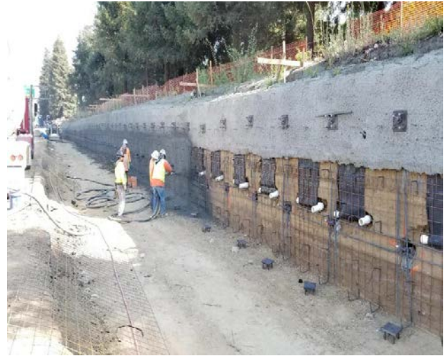
Shotcrete placement at soil nail wall, Hacienda Overcrossing
