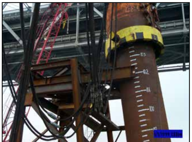
Battered Pile Installation Demonstration
