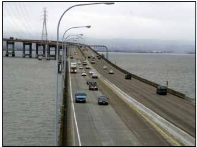
High-Rise Section of San Mateo-Hayward Bridge
