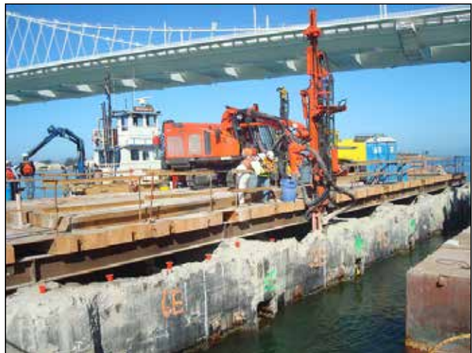
E3 Foundation Blast Hole Drilling In Progress
