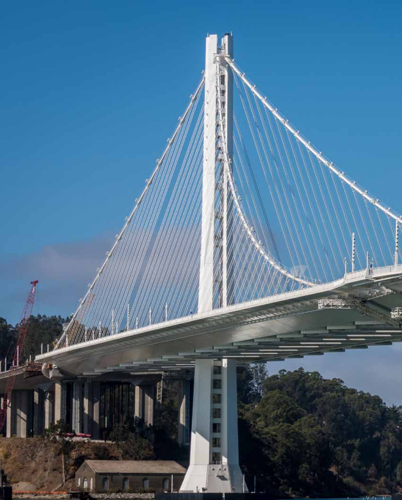
View from the Bay of the San Francisco-Oakland Bay Bridge Self-Anchored Suspension Bridge
