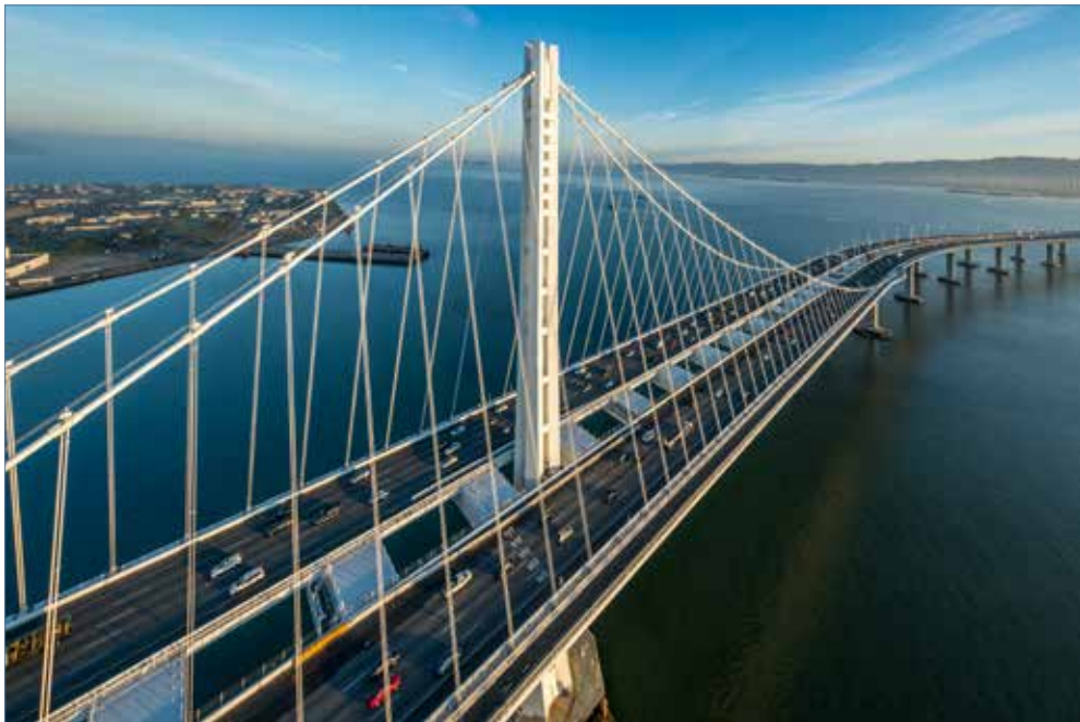
The Self-Anchored Suspension Bridge Span Looking east toward Oakland
