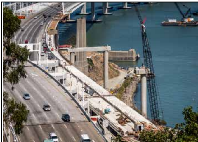
Bike/Pedestrian Pathway Construction Progress
