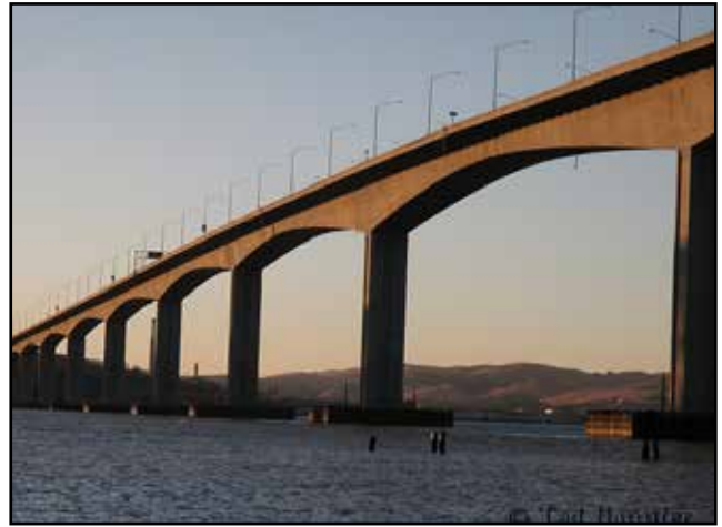
The New Congressman George Miller Bridge (New Benicia-Martinez Bridge)
