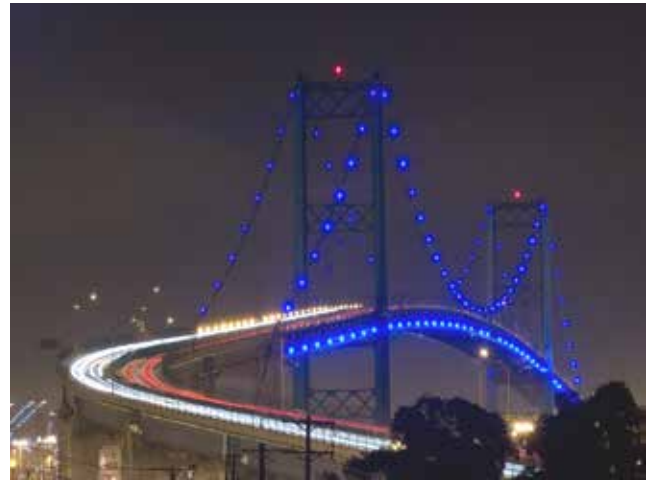
Los Angeles-Vincent Thomas Bridge
