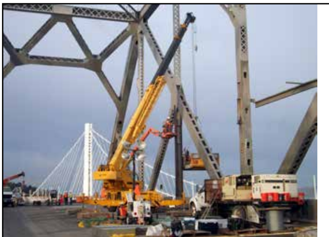
Former Superstructure Dismantling Progress
