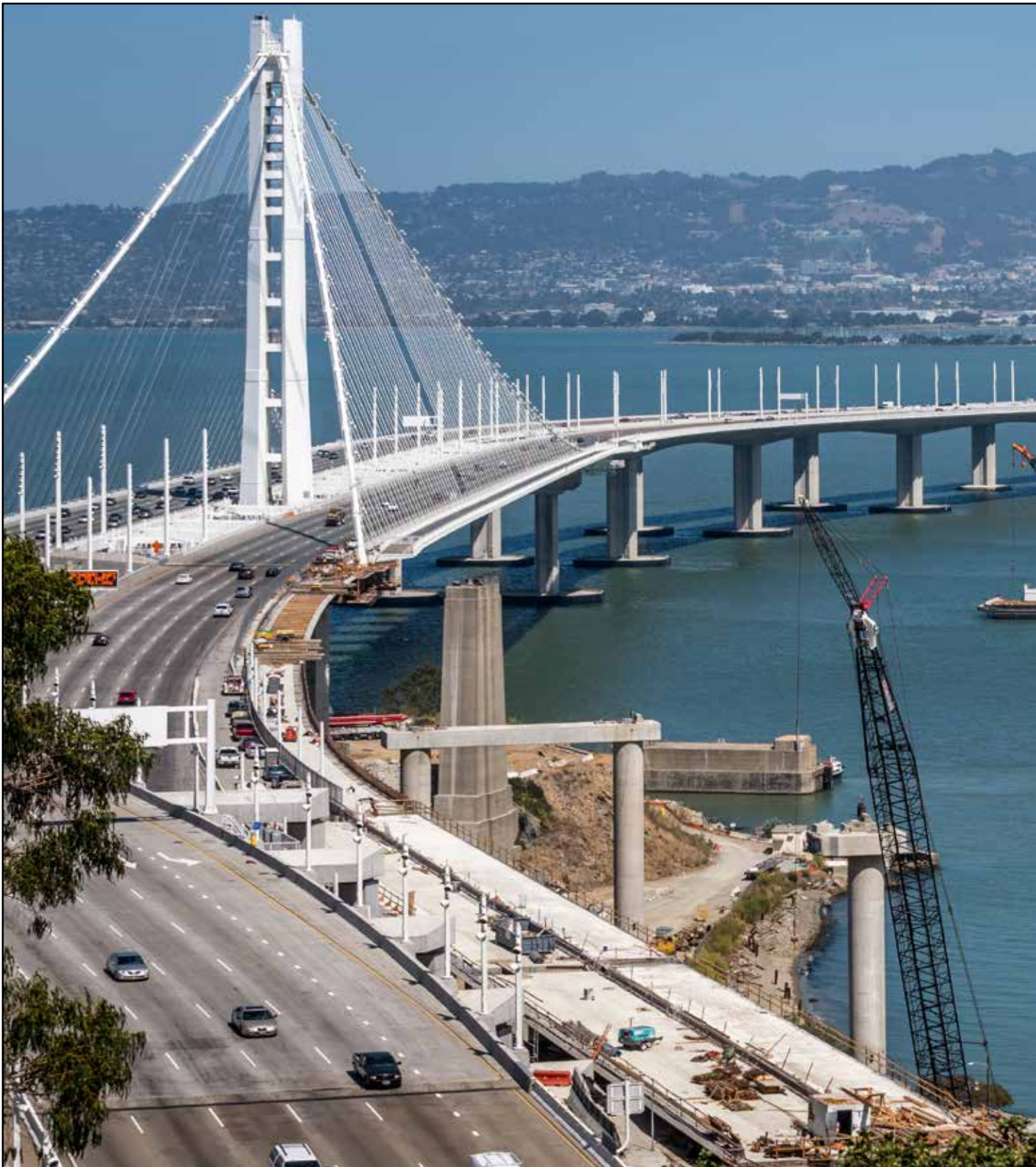
Yerba Buena Island Transition Structures Demolition Progress on right with the New Self-Anchored Suspension Span of the San Francisco-Oakland Bay Bridge on left Looking east toward Oakland
