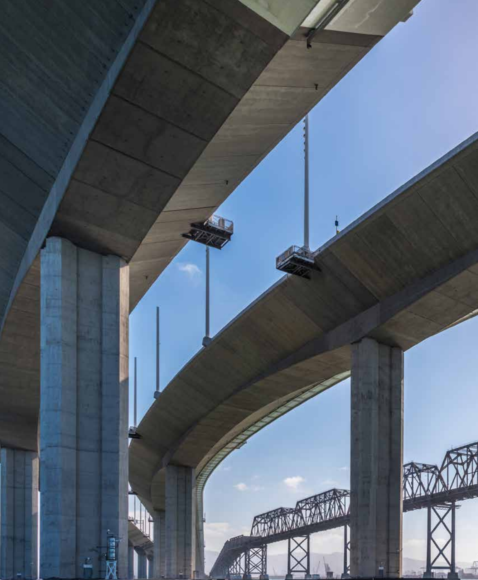
The Skyway of the New San Francisco-Oakland Bay Bridge from the Surface of the Bay with the Dismantling of the Former Bridge on the right
