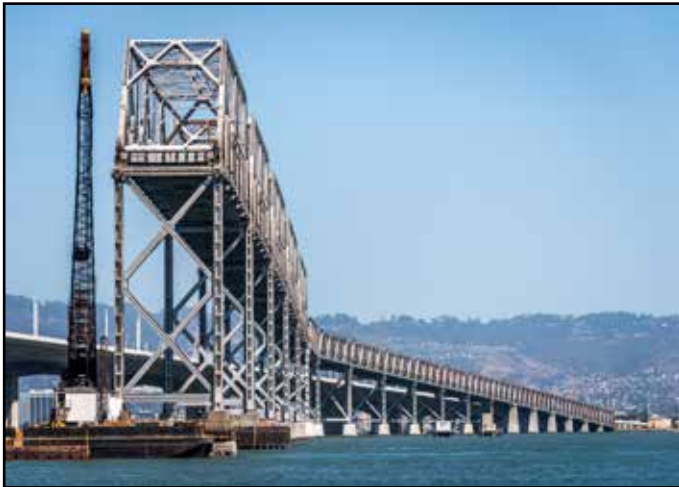
Dismantling Progress on the Former San Francisco-Oakland Bay Bridge
