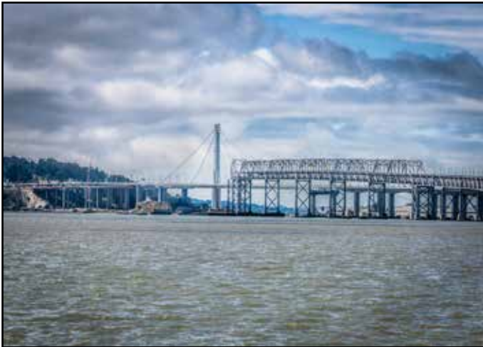
Former Superstructure Dismantling Progress
