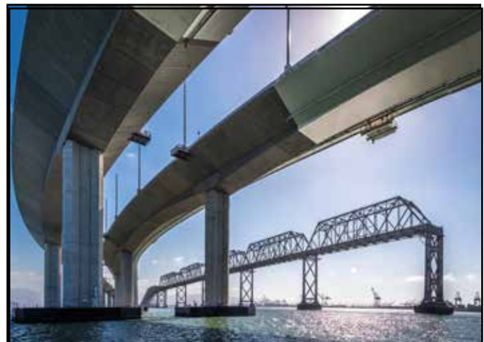
The New Skyway on left and Dismantling of Former Bridge on right
