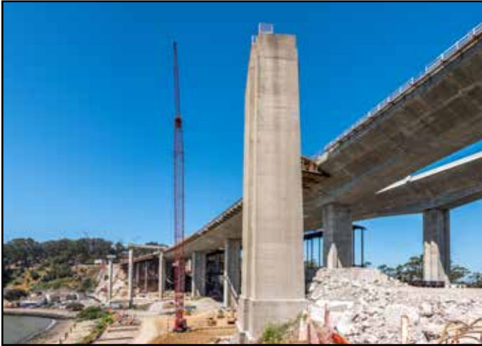
Former Superstructure Dismantling Progress
