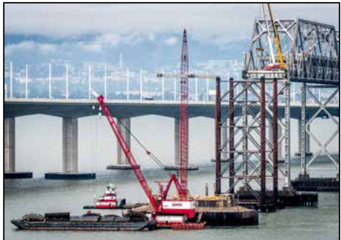
Dismantling Progress of the Old San Francisco-Oakland Bay Bridge
