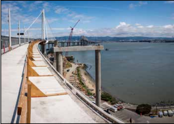
Self-Anchored Suspension Bridge Bike Path Construction
