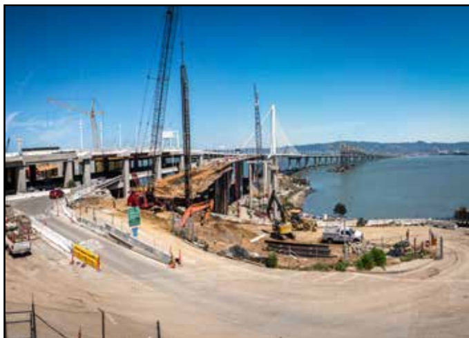
On-Ramp and Pedestrian/Bike Pathway Progress
