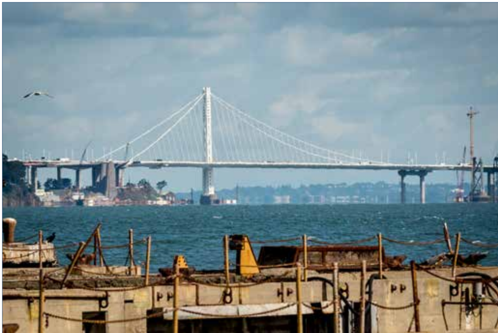
The Self-Anchored Suspension Bridge Span
