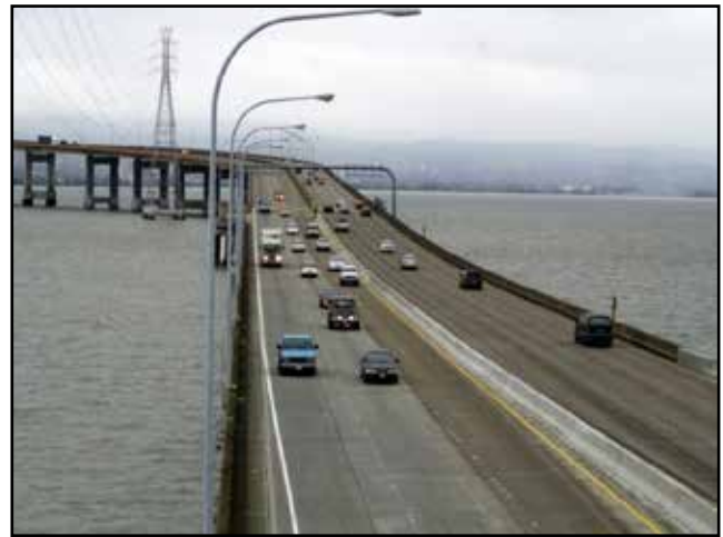
High-Rise Section of San Mateo-Hayward Bridge
