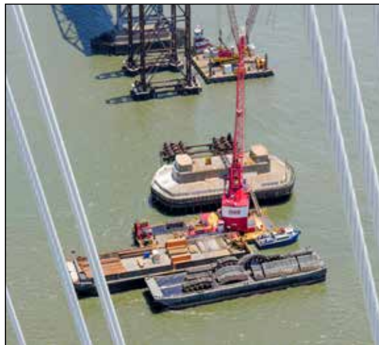
E3 Foundation Removal
