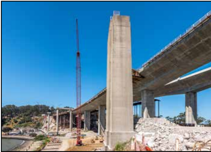
Superstructure Dismantling Progress
