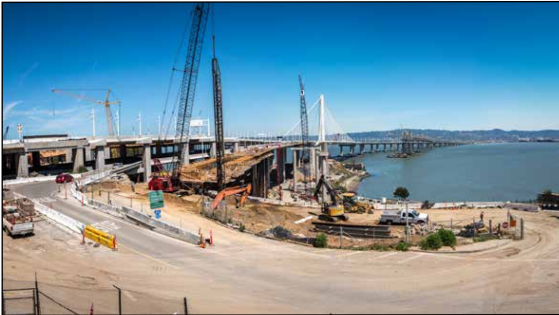
Eastern Span of the San Francisco-Oakland Bay Bridge Bicycle/Pedestrian Path and Ramp Construction in Progress
