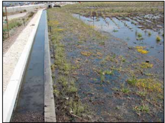
Stormwater Retention Basin
