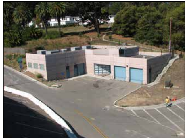
New YBI Electrical Substation
