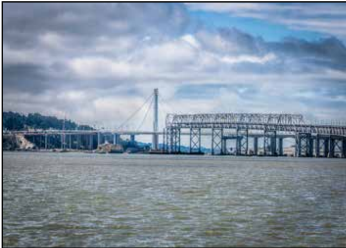
Superstructure Dismantling Progress
