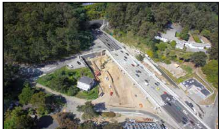
West Tie-In Phase # 1 Rolled in on Labor Day Weekend 2007
