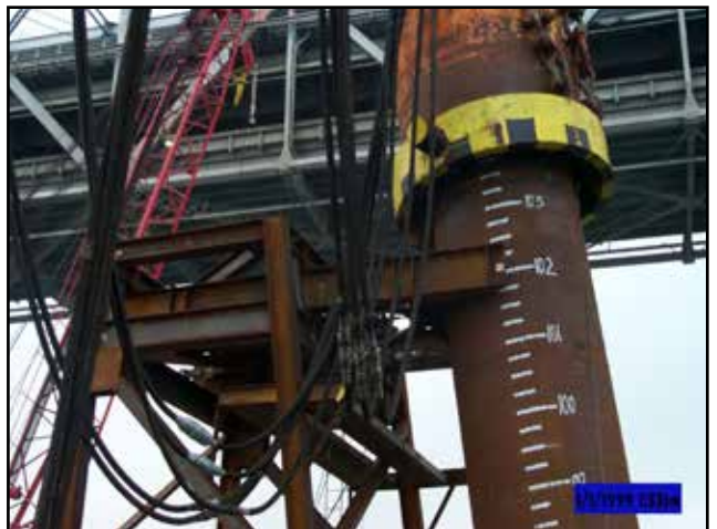
Battered Pile Installation Demonstration
