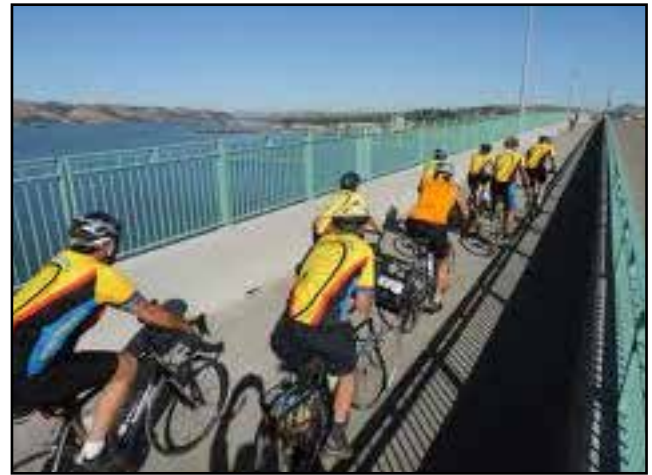
Benicia-Martinez Bridge Bicycle/Pedestrian Path
