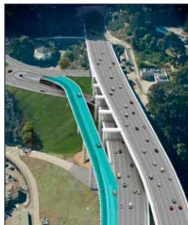
Birds-Eye View Simulation of the Yerba Buena Island Transition Structures and the New San Francisco-Oakland Bay Bridge Eastbound On Ramp and Bicycle Path after Dismantling of the Existing Structure
